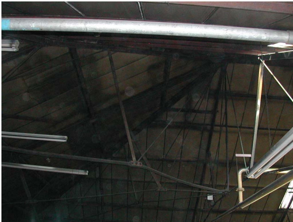
Half-trusses at hipped end of bay 1
