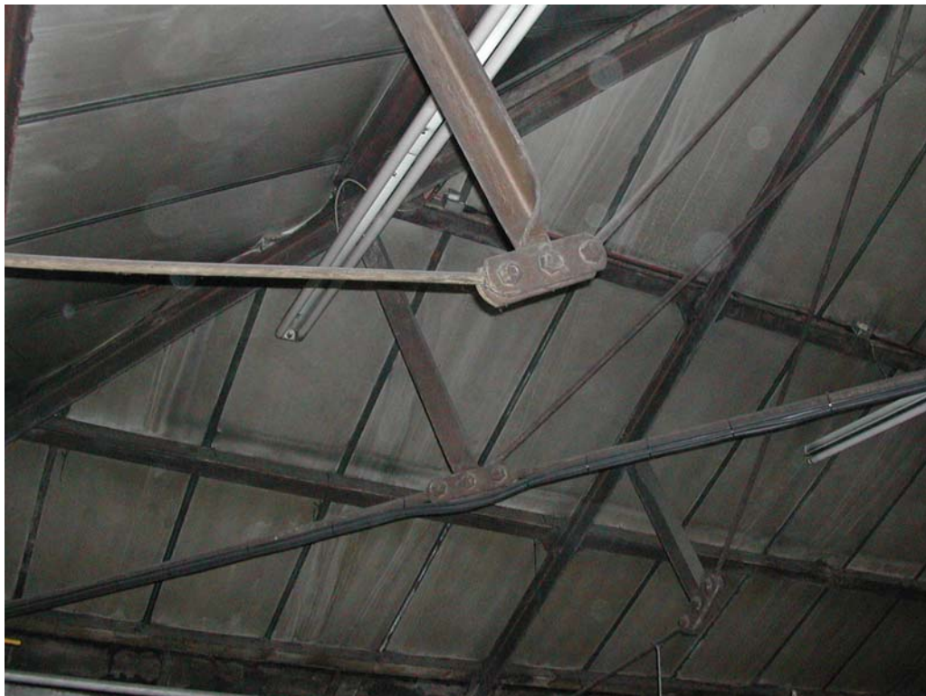
Half-truss and braced principle rafters at hipped end of bay 1.
